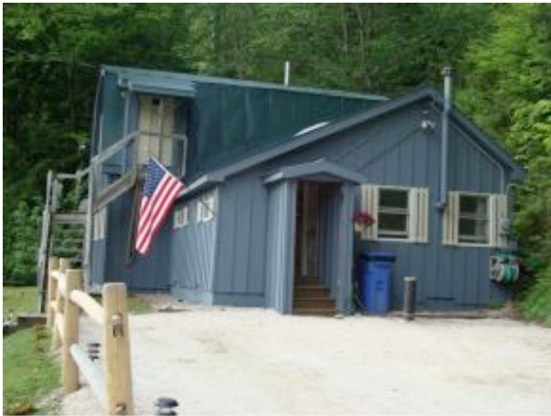
View from re surfaced driveway
